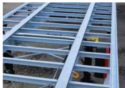
Welded structural steel platform with I-beams spaced at 400 mm intervals
